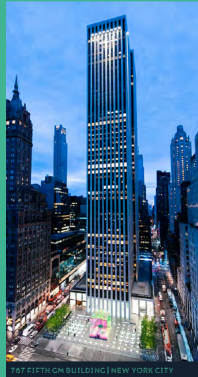
767 FIFTH GM BUILDING | NEW YORK CITY
